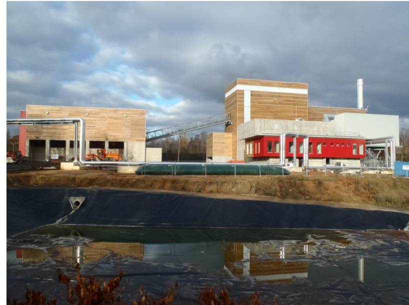
Picture : Forbach (6.4MWe ; 24 MWth)
